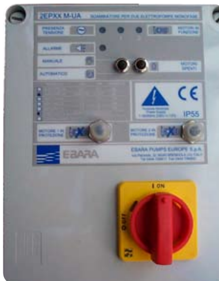
Control panel for dual pumps
