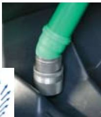
Multisiphon trapped overflow with verimin guard and backflow prevention
