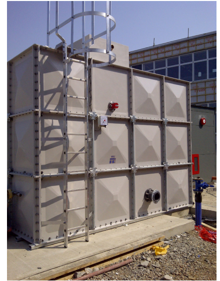
Internal and external ladders can be supplied as required
