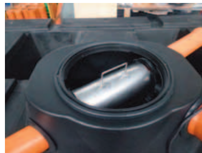
The compact design allows the filter to be easily fitted into the access shaft of an underground tank.
