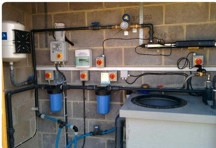
Break tank with sediment filters & UV disinfection
